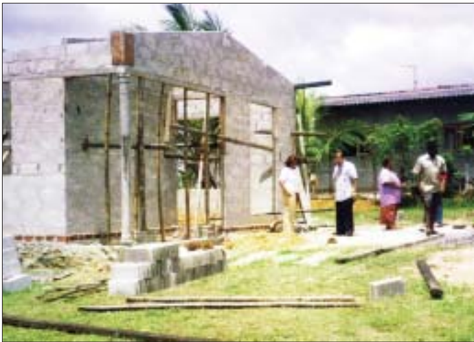
Houses under construction
